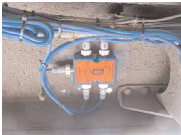
Example installation of 4 way junction box
